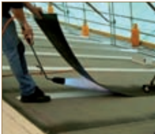
Rolled roof installation
